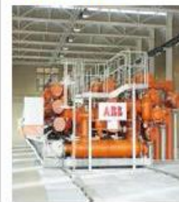
Compact 420 kV substation
