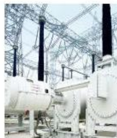
Ultra high- voltage 1100 kV GIS substation
