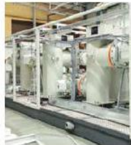
145 kV GIS in prefabricated housing
