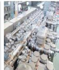
Eco-GIS substation
